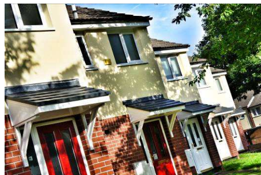
Secure by Design windows and doors, and external insulating cladding on homes. Cranwell Road, Strelley
